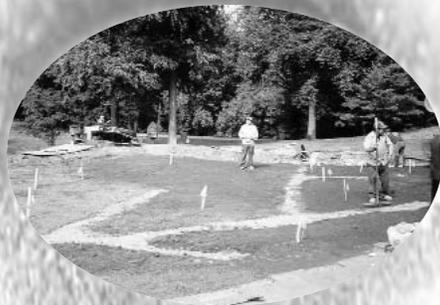
*Drainage is installed with pea gravel, which is even with the subgrade.*
